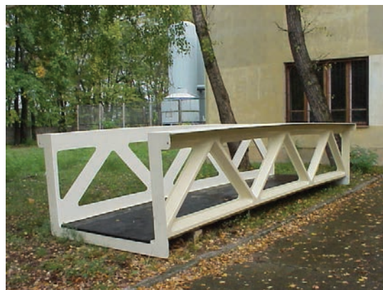
Fig. 1. The prototype of the composite footbridge section [3]
