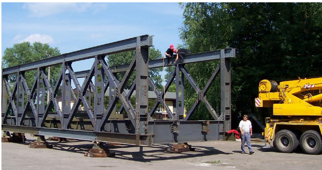
Fig. 1. The ŽM 16 bridge structure at the training base of the Ministry of Transport of the Czech Republic
