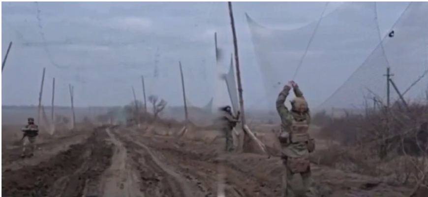
Russian troops build a two-kilometer mesh net "tunnel" in early 2025 to protect against Ukrainian FPV drones. In theory, FPV drones on their final attack trajectory will get entangled in the net or go off course. Screenshot from X
